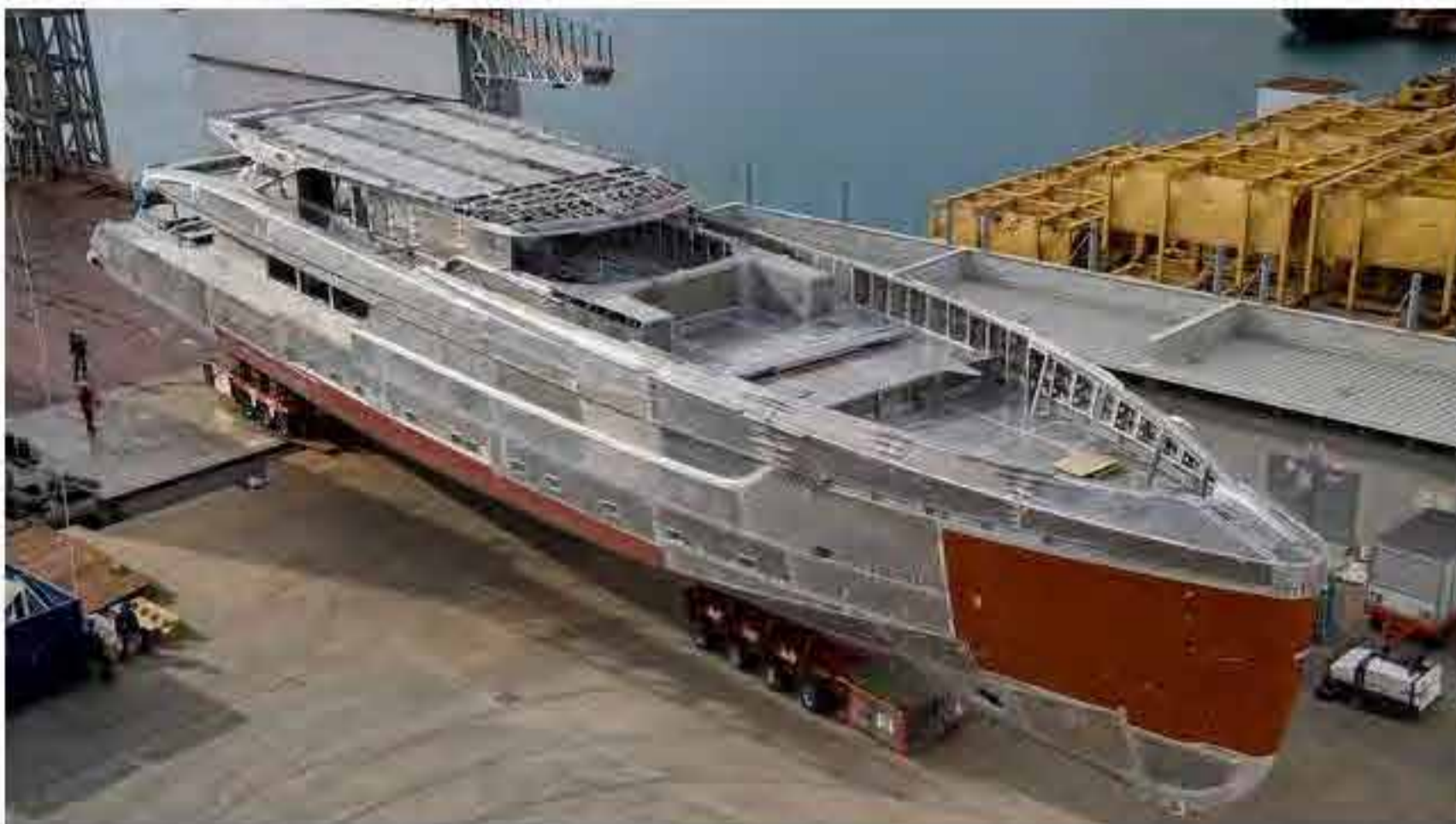
The aluminium construction of S501 is complete and the yacht has been moved to the completion shed
